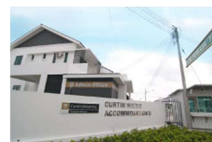
Curtin Water-II Accommodations
